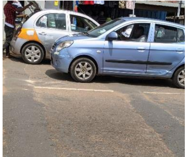
Figure 3-7: Speed hump on a local road
