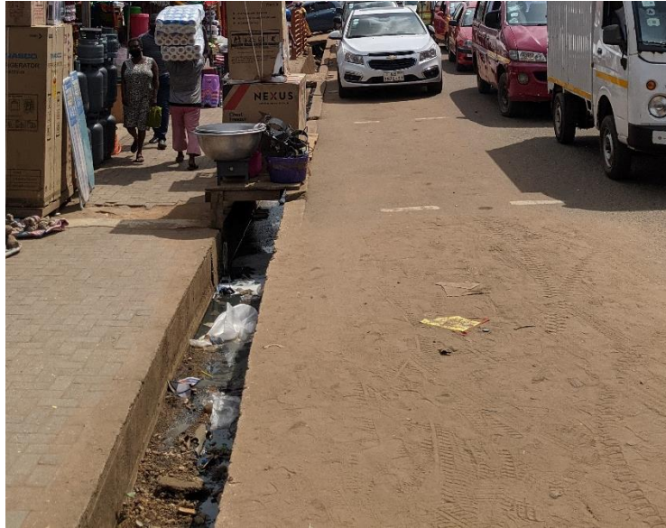
Figure 3-13: Open drains turned into garbage bins
